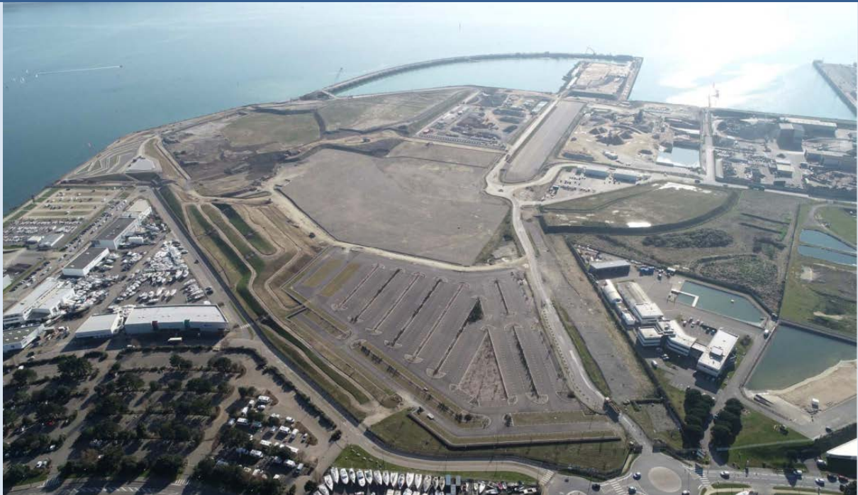
Figure 10-4: Partially Complete Marine Works at Port of Brest 2019 [48]
