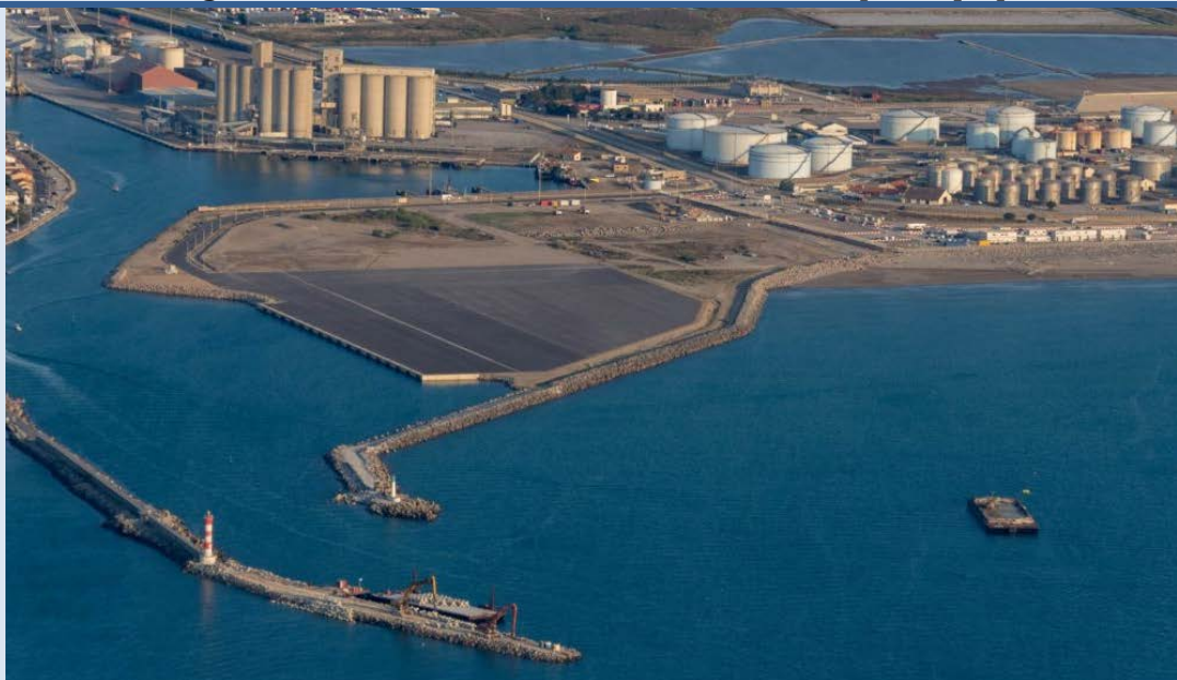
Figure 10-2: Completed Heavy Lift Quayside and Partially Complete Breakwaters [44]
